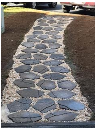
New Sidewalk for building 2
